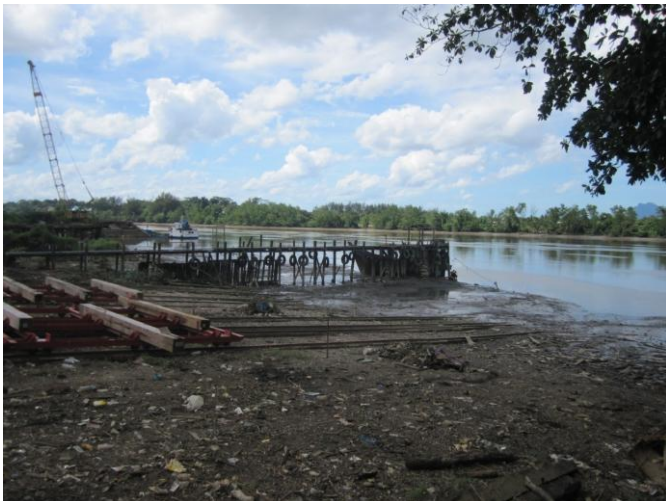
Figure 3: Jetties and Riverbank Conditions in Bintawa
