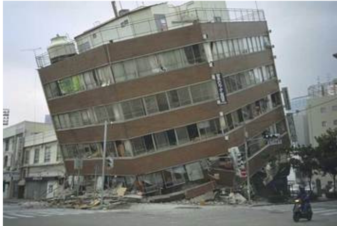
Figure 1.1: A collapsed building in Japan's 1995 Kobe Earthquake
