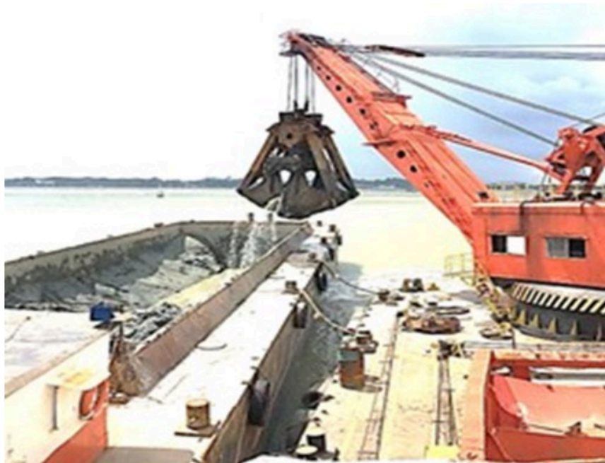
Fig. 1. Clamshell dredger (Johor, Malaysia)
