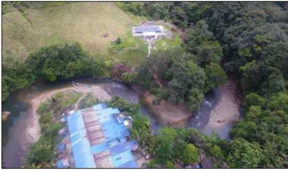
Fig. 1. Picture of the Rumah Bada Longhouse and its solar PV systems [6].
