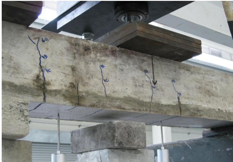
Figure 5: Cracking pattern of ferrocement strengthened beam
