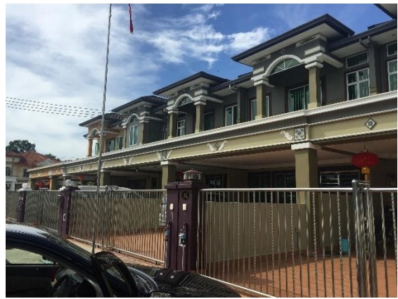
Figure B – 9(b): Residential Area 9
