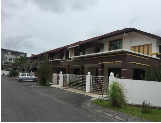
Figure B – 7(a): Residential Area 7
