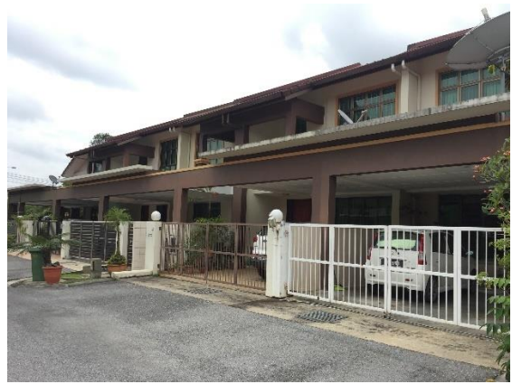
Figure B – 7(b): Residential Area 7
