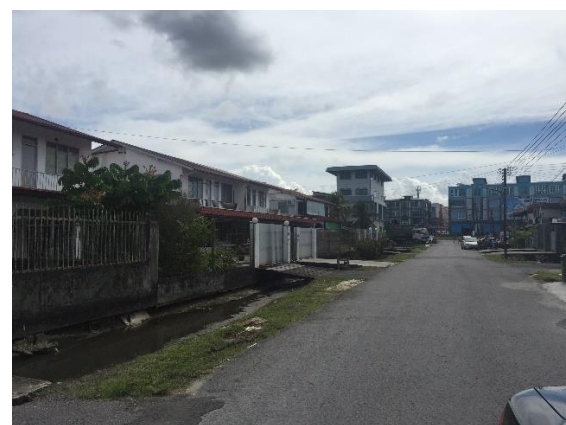
Figure B – 10(b): Residential Area 10
