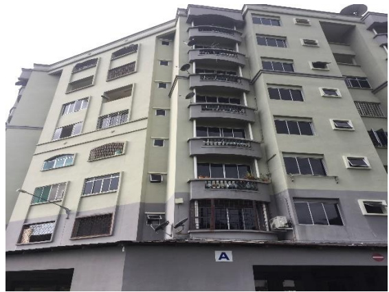
Figure B – 8(b): Residential Area 8
