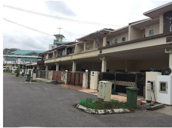
Figure B – 1(b): Residential Area 1
