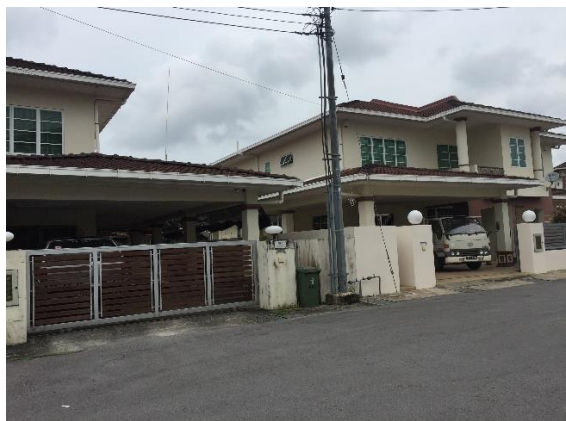
Figure B – 2(b): Residential Area 2
