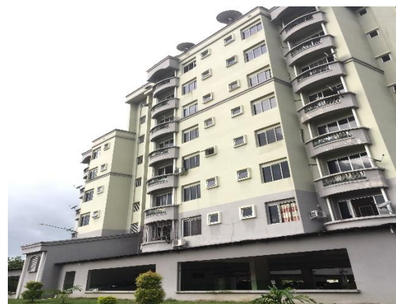
Figure B – 8(c): Residential Area 8
