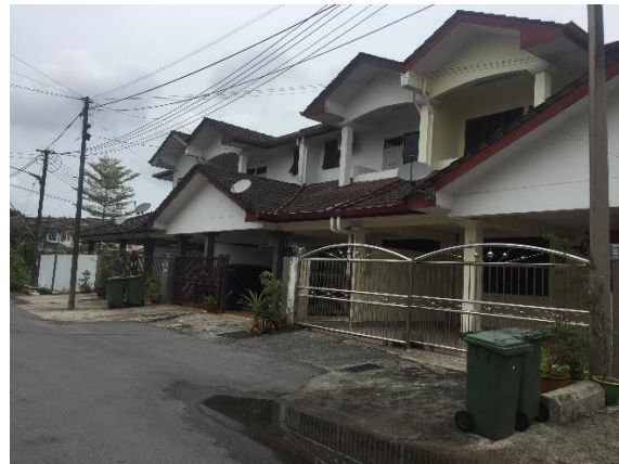
Figure B – 4(b): Residential Area 4
