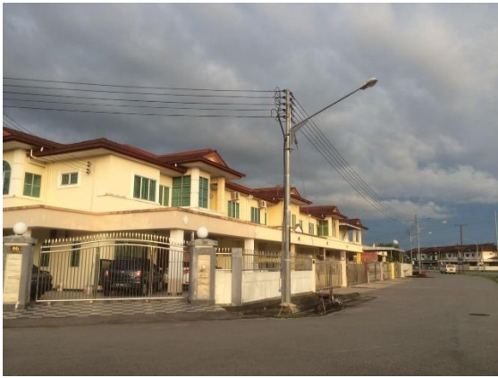
Figure B – 9(c): Residential Area 9
