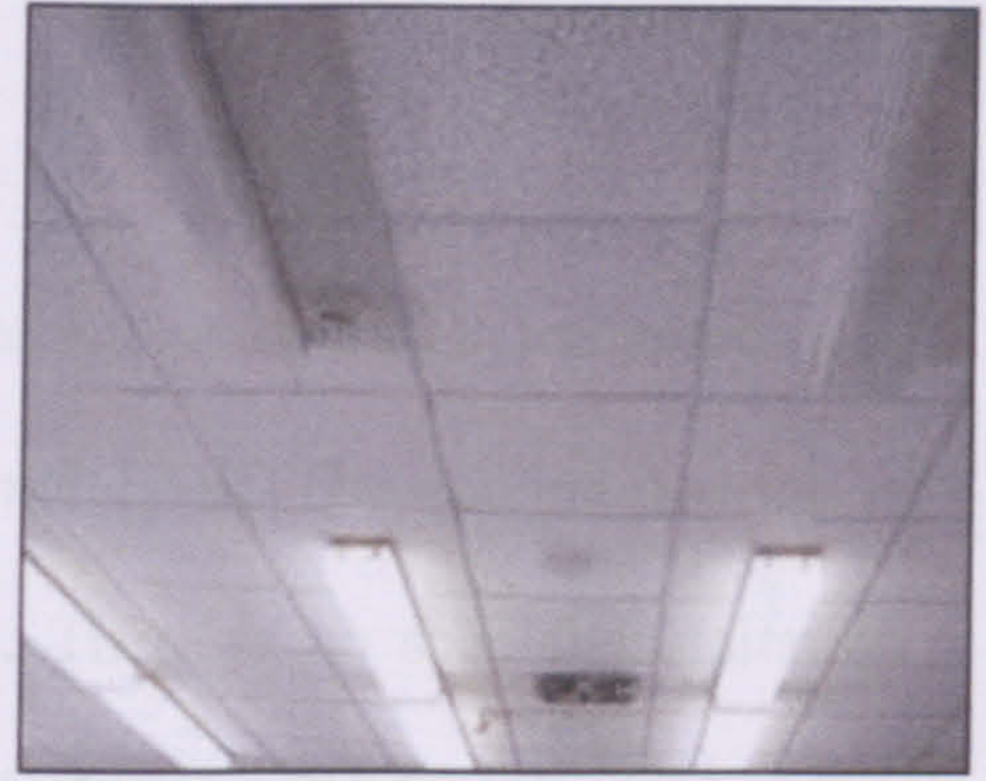
Figure 2.2: Drop ceiling or suspended ceiling
