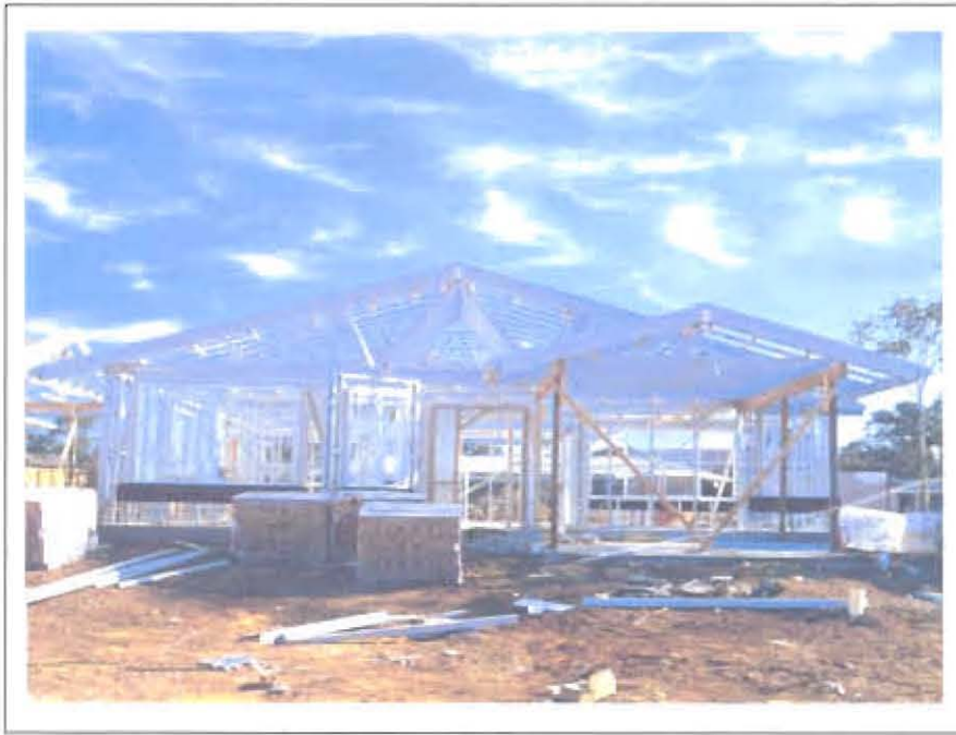
Figure 1.1 A residential house built with cold-formed steel (Source: BHPSteel 2002)
