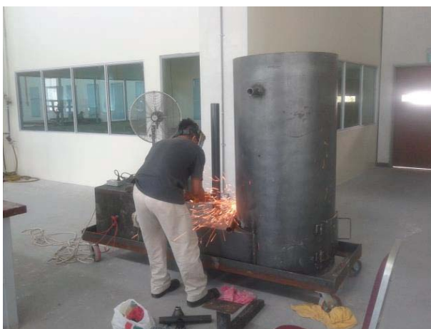
Figure L 57: Cutting process for pipe connection
