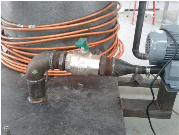
Figure L 67: Pipe and 1.5-inch ball valve at the blower 2 is welded
