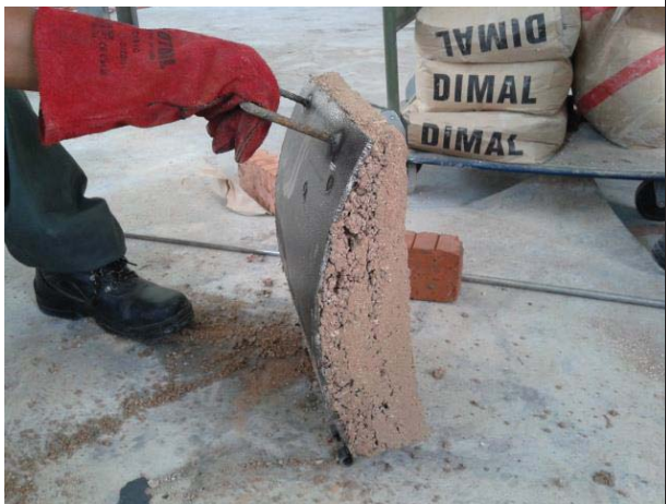
Figure L 31: Refractory door at pyrolysis chamber is formed
