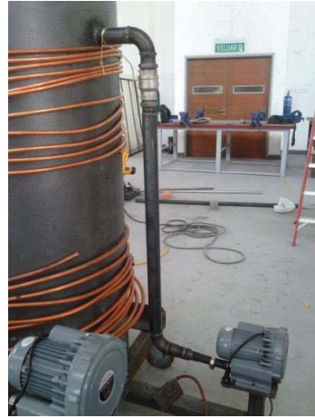
Figure L 66: Pipe and 1.5-inch ball valve at the blower 1 is welded
