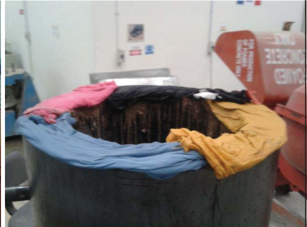
Figure L 42: Refractory surface is covered with wetted cloth for 24 hours
