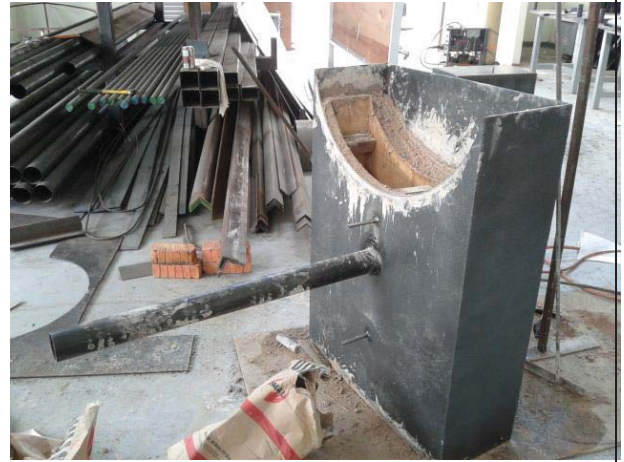
Figure L 26: Refractory is filled in the tar removal chamber framework (left for 24 hours)
