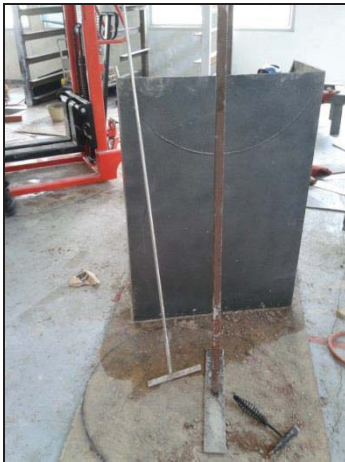
Figure L 25: Customized tools to compact the refractory
