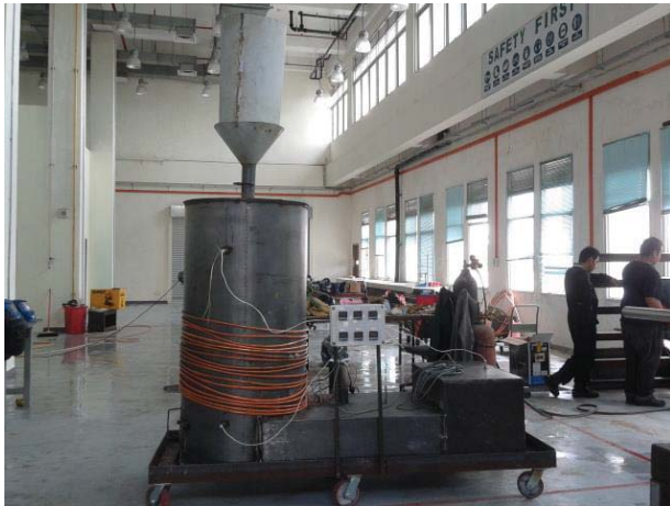
Figure L 77: Fabrication of B2H is completed
