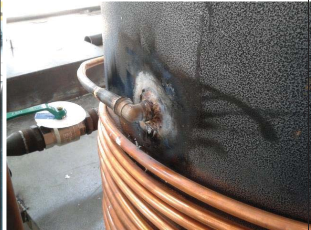
Figure L 74: Copper tube is fitted with a copper jointer
