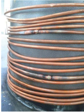
Figure L 71: Copper tube is welded
