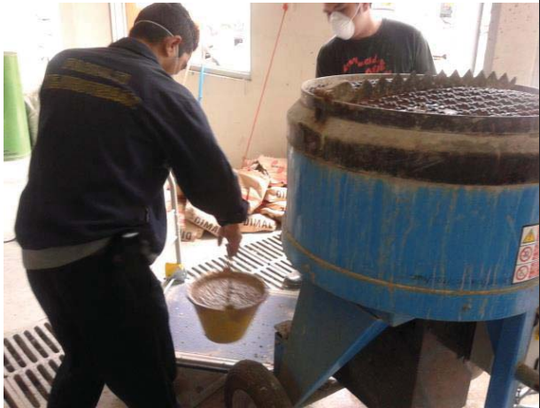
Figure L 35: Mixed refractory produced by concrete machine
