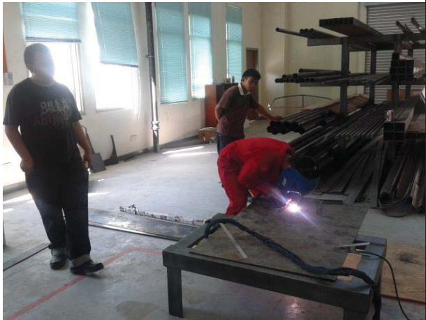
Figure L 13: Plasma cutting 6-mm mild steel for fuel gas-to-heat energy conversion chamber
