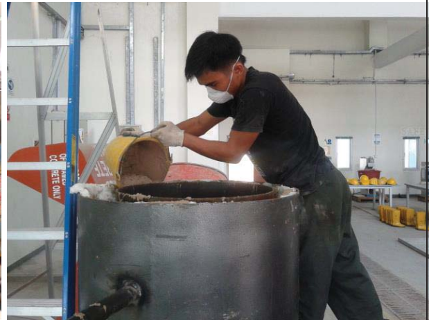
Figure L 36: Filling the mixed refractory into the pyrolysis chamber framework
