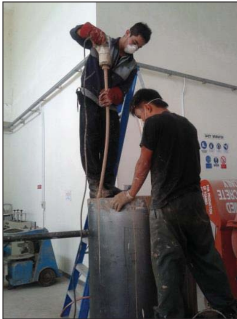
Figure 3.5: Refractory is compact with concrete vibrator to avoid void form
