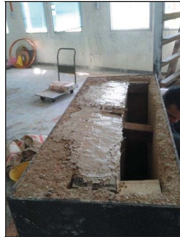
Figure L 30: Inclined is built inside the tar removal chamber
