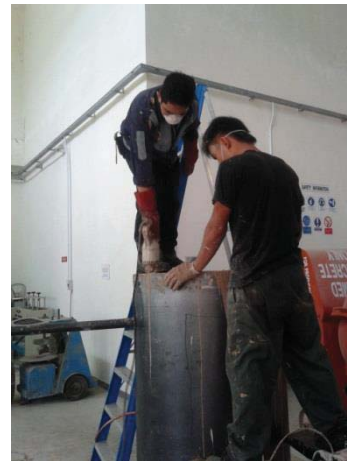
Figure L 38: Process of working with concrete vibrator
