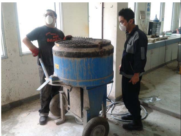
Figure L 33: Concrete mixer machine is used for mixing refractory
