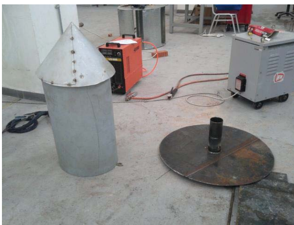
Figure L 63: Completion of hopper and B2H cover
