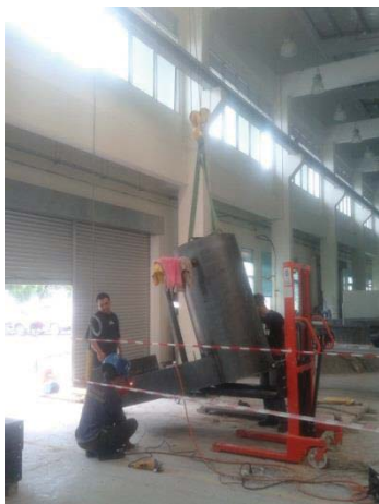
Figure L 51: Positioning the B2H by overhead crane for welding
