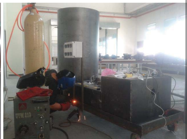
Figure L 58: Installing thermocouple indicator box and its stand
