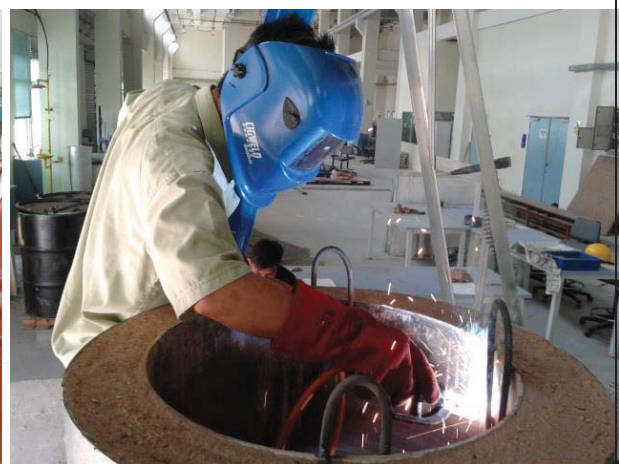
Figure L 46: Welding "U" bars inside the pyrolysis chamber for lifting work
