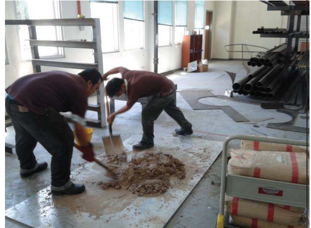
Figure L 24: Refractory is mixing with water accordingly
