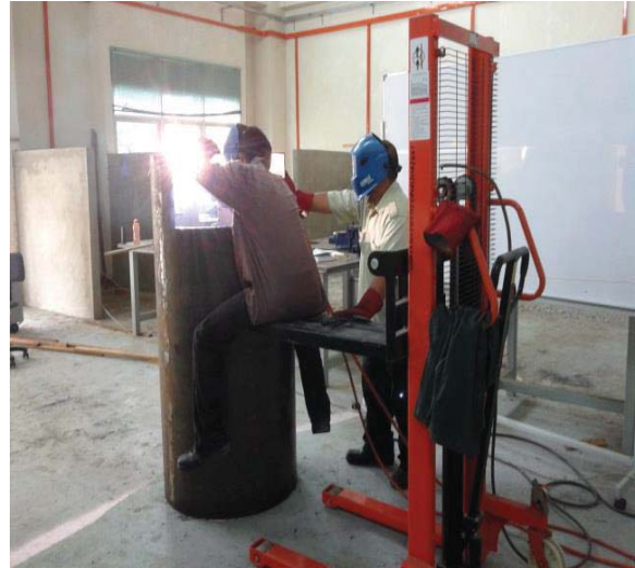
Figure L 2: Welding the base of pyrolysis from inside
