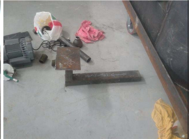
Figure L 54: Blower stand is fabricated
