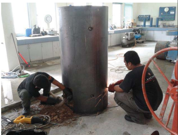
Figure L 45: Chiseling and cutting work on pyrolysis chamber
