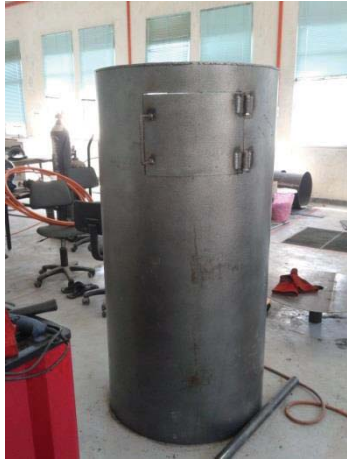
Figure L 17: Pyrolysis chamber door is welded
