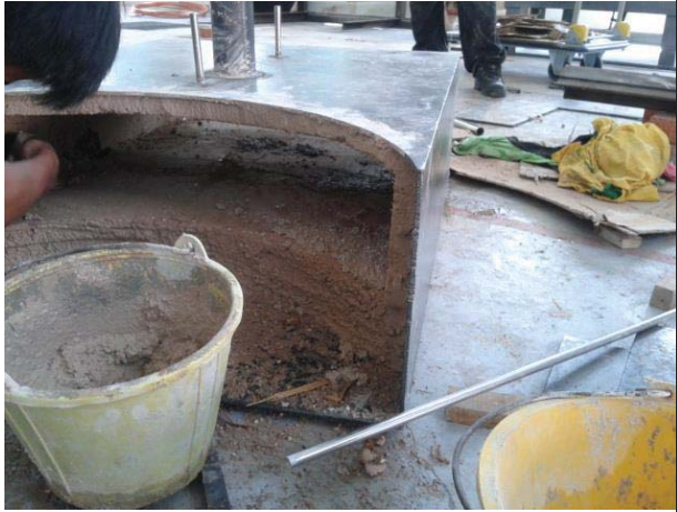
Figure L 29: Refilled the refractory in the void found
