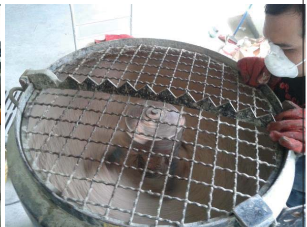
Figure L 34: Top view on the working concrete mixer machine
