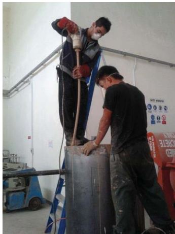
Figure L 37: Refractory is compact with concrete vibrator to avoid void form
