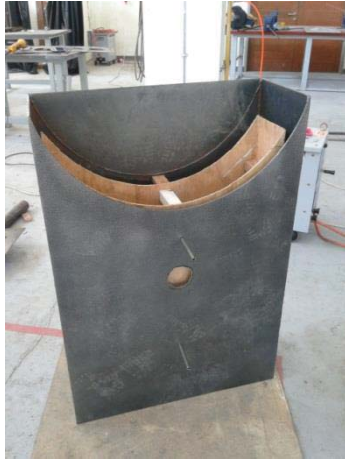
Figure L 23: Wooden framework is formed at tar removal chamber before fill in refractory
