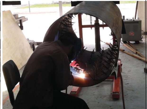
Figure L 4: Welding "V" anchor bar inside the pyrolysis chamber
