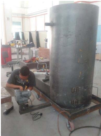
Figure L 55: Installing the blower 1 on the blower stand
