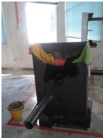
Figure L 27: Wet cloth is covered the surface area of refractory in tar removal chamber for 24 hours
