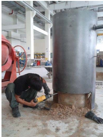
Figure L 43: Chiseled the extra refractory by chisel machine
