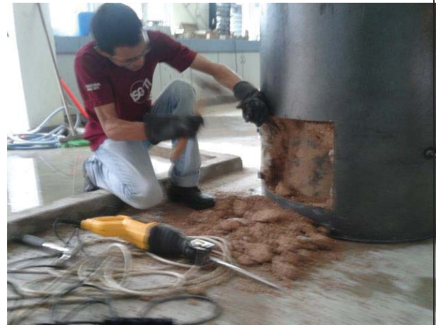
Figure L 44: Chiseled the extra refractory by hammer and chisel
