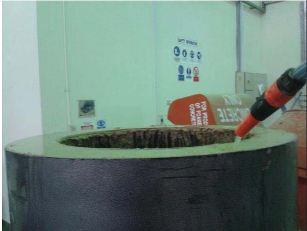
Figure L 41: Refractory surface is wetted for curing process
