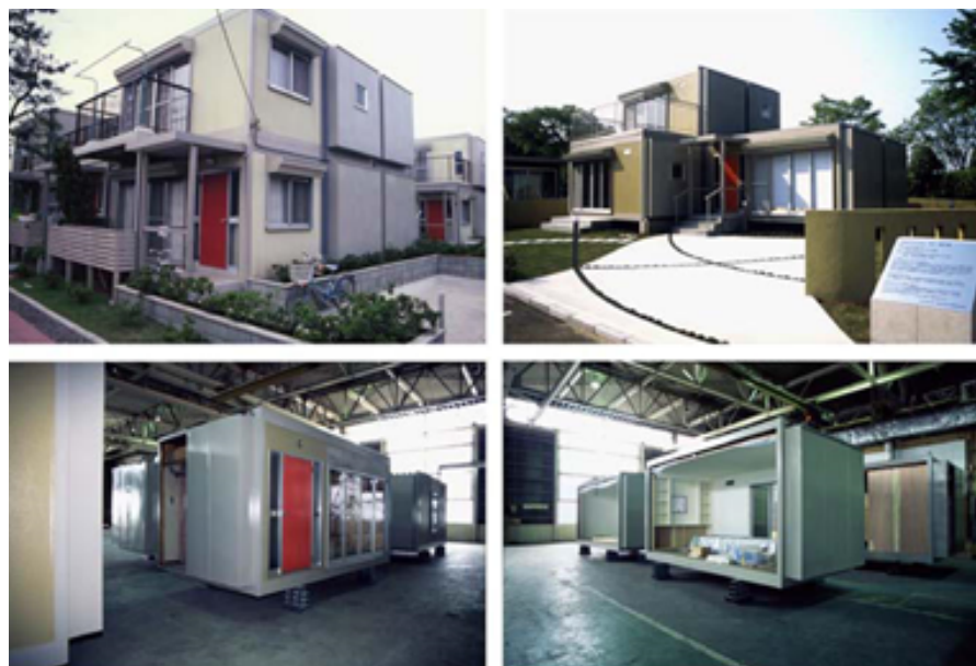
FIGURE 3: Sekisui Heim's Model M1 Reached Production of 3000 Building/Year for Several Years (Linner, 2012)
