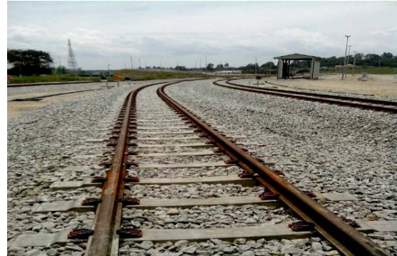
Fig. 1 Ballasted track (Depot KTM Gemas Malaysia, 2013)
