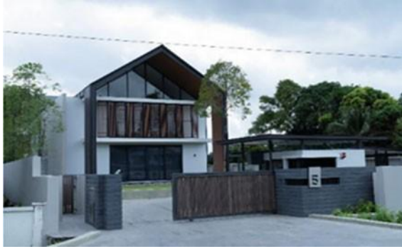
Fig. 2 Shows the security guard’s house before entering A House
