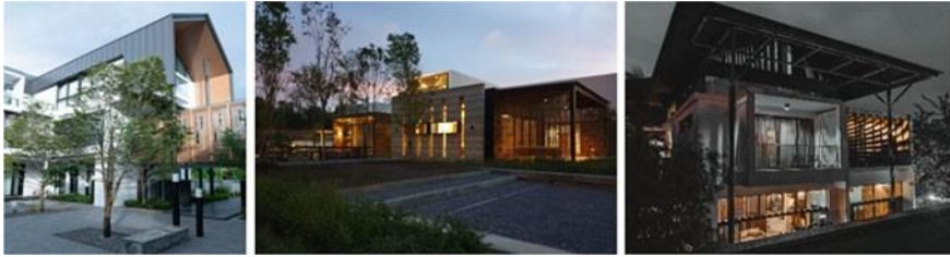
Fig. 5 (Left) A House with a cantilever seam roof in which the roofing edge extends beyond the house’s exterior walls. (Middle) B House with a facade sunscreen attached to the exterior of the house. (Right) C House with a big canopy roof over the external faces of the house that provides an aesthetic form of shading from the hot climate
