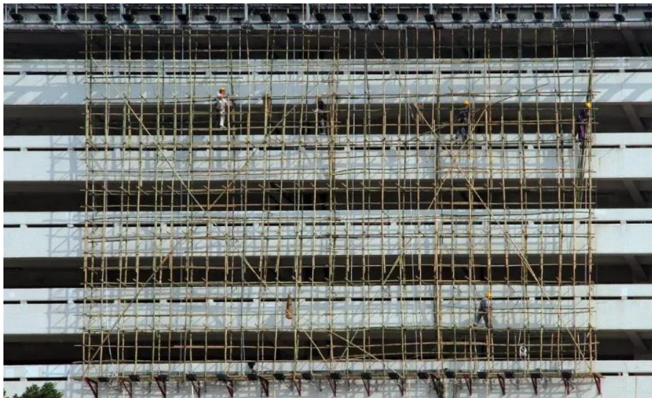
Fig. 2. Bamboo scaffolding (Neumann 2020)
