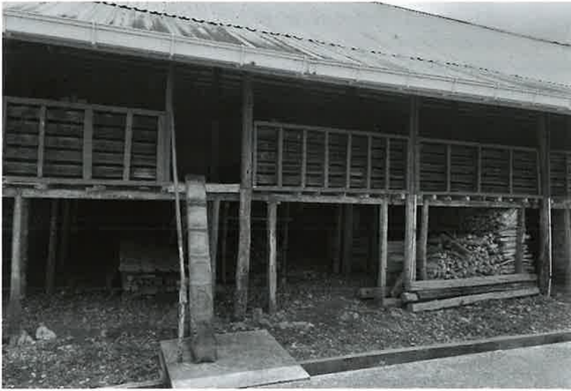
Figure 3. A hybrid vernacular longhouse in Mongkos, featuring a notched log staircase and zinc roof, 2023, Azmah Arzmi.
