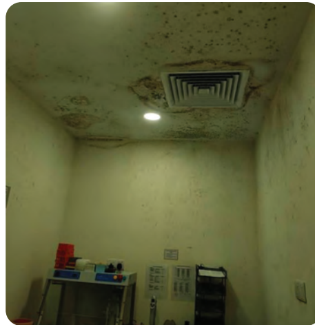
Figure 2. Dark patches of mould growth are visible on the surfaces.
