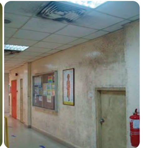
Figure 2. Dark patches of mould growth are visible on the surfaces.
