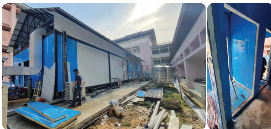
Figure 6. PU panel insulative walls.
