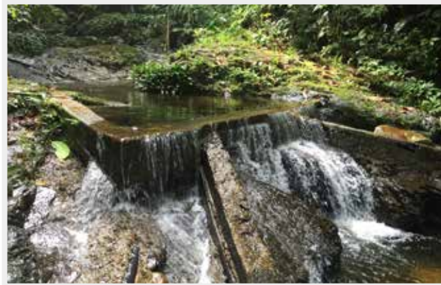
Figure 23.3. Villagers in Bong rely on this water impoundment in order to obtain their daily source of potable water. Previously, they used to depend on the rainwater harvesting system that is no longer used prior to the introduction of the current gravity-fed system.
