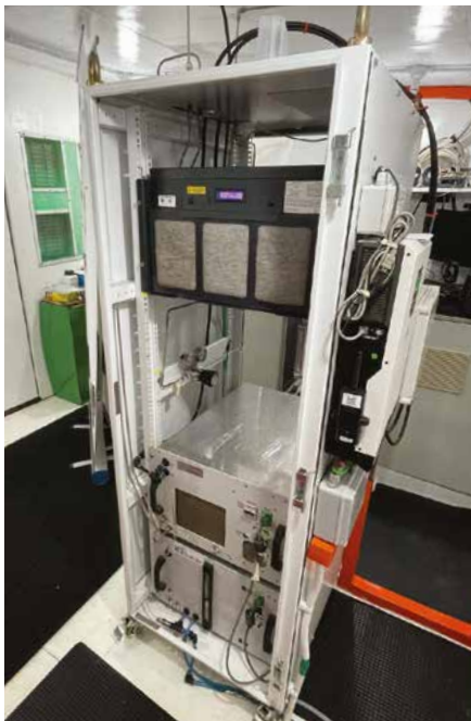
Figures 6A and 6B: The hydrogen fuel cell system (left) linked to a solar PV system to generate 'green' electrical energy in a rural healthcare clinic in Borneo Sarawak.
