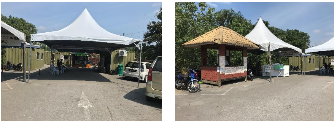
Figure 4.1: Bako Boat Terminal Before Renovation in 2019: (1) The waiting area, Bako National Park ticketing booth and Bako Boat Association (Old) boat ticket service counter; (2) Bako Boat Association (New) boat ticket service counter
