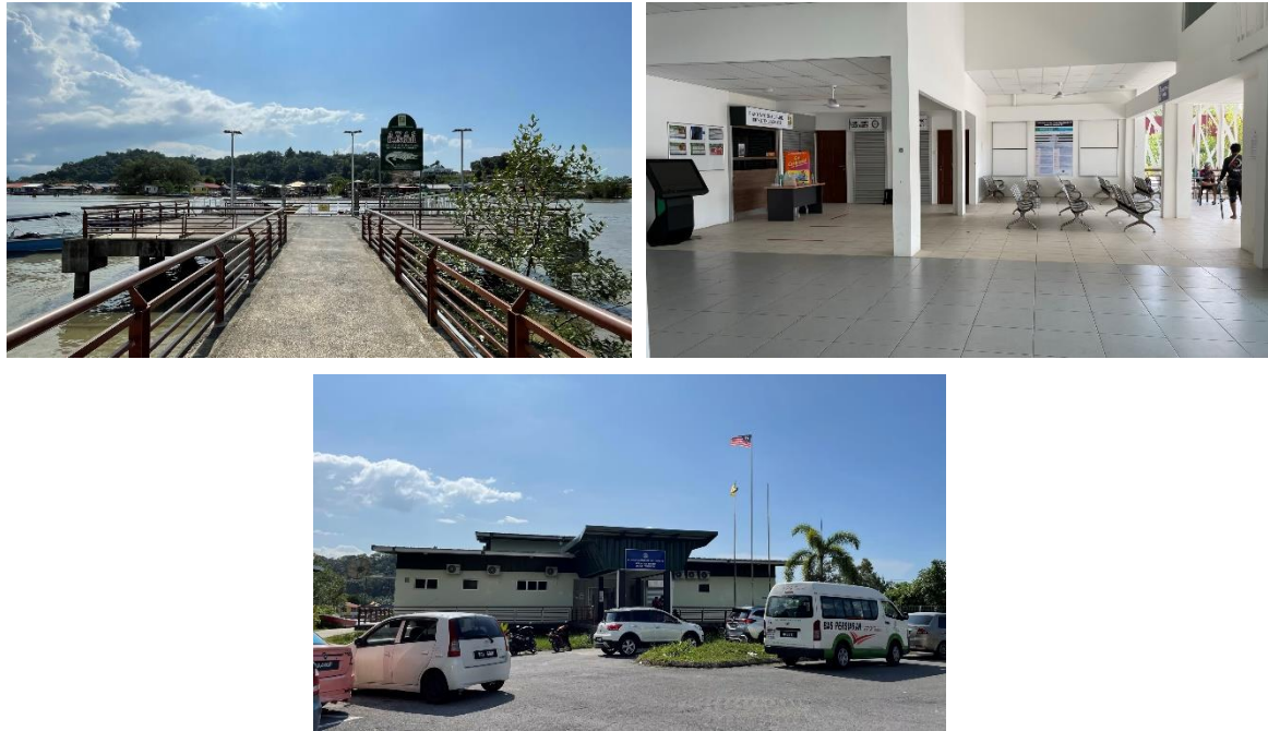
Figure 4.2: Bako Boat Terminal After Renovation: (1) Jetty to the boat; (2) Waiting area, Bako National Park ticketing booth and boat ticket service counter; (3) Entrance of jetty to Bako National Park
