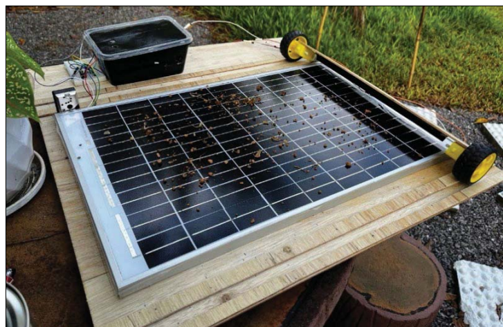
Figure 4.2: Solar Panels with Dust Accumulation
