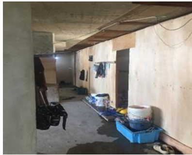
Fig. 2. Construction Site A makeshift workers' quarters setup made of plywood partition boards.
