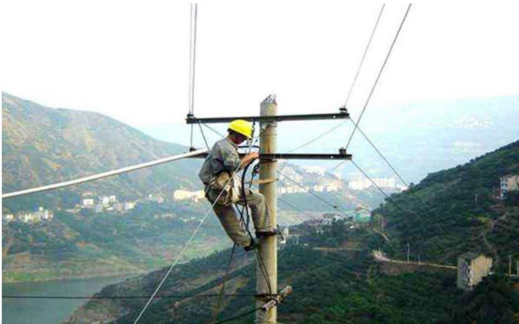
Figure 1.1: Manual inspection of power line [8]
