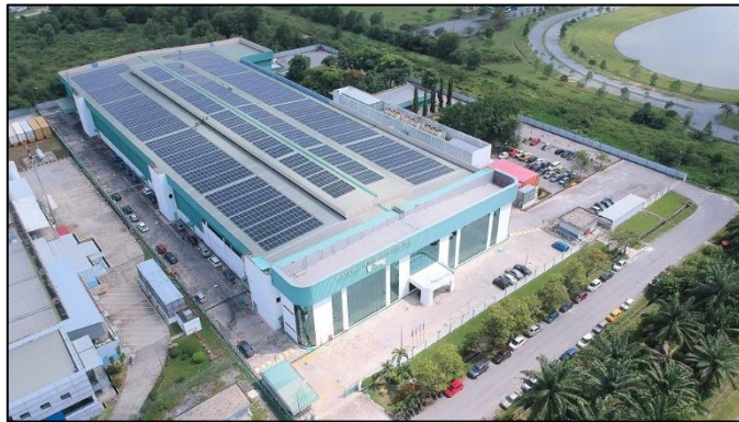
Figure 1.5: Rooftop solar PV at Mölnlycke in Malaysia [13].
