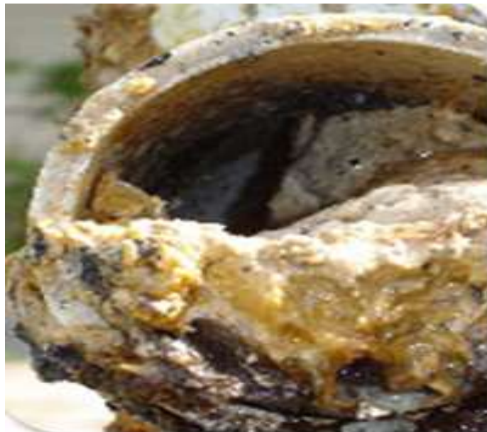
Figure 2.3. Buildup of FOG in the grease trap. (Adapted from Martin, 2017).
