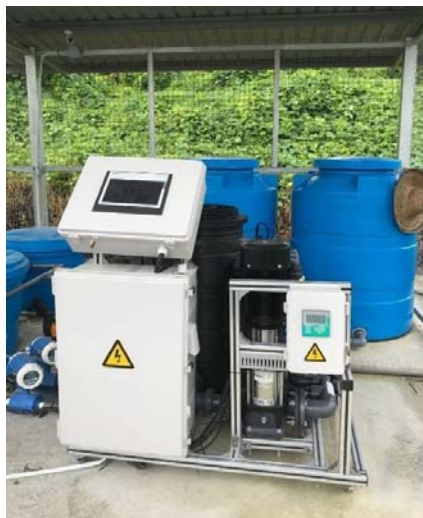
Figure 2.8 Automated fertigation system to control fertilizer content and irrigation and storage tanks. (Photo taken at Agriculture Research Centre, Semongok.)
