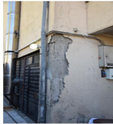
d) Building B
