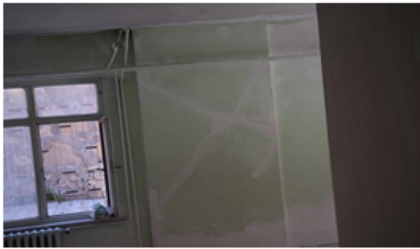
a) Building A
