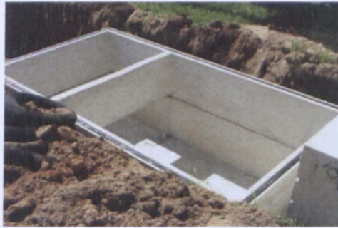
Figure 2.5: Typical Underground Water Tank ( www.precast.org ).
