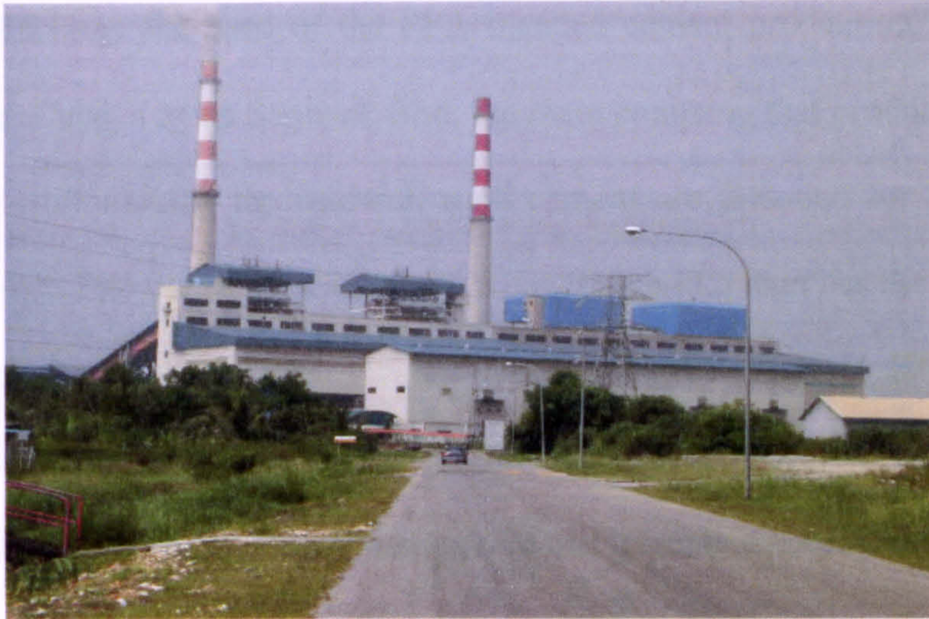
Figure 1.2 Sejingkat Power Station
