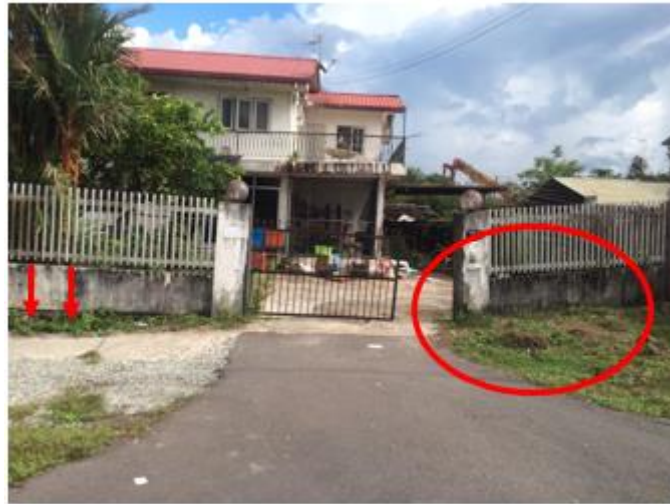
Figure 1.3. Settlement at housing area located at Jalan Oya, Sibul.
