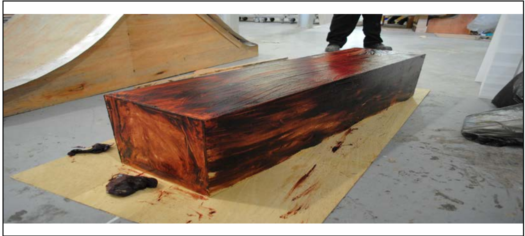
Figure 3.8: Formwork with Grease
