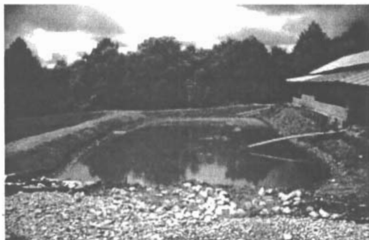
Figure 1: A typical pig waste lagoon which is found in Gedong, Sarawak. According to the correspond farmer, the pond depth is around 5 to 6 feet. This lagoon might be characterized as a facultative lagoon.
