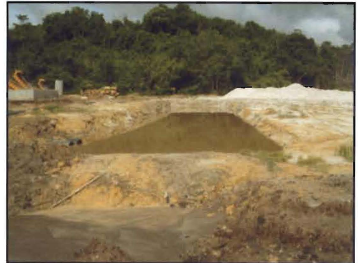
Plate 15: Example of a Sedimentation Pond (Courtesy of PSS Resources Sdn Bhd)
