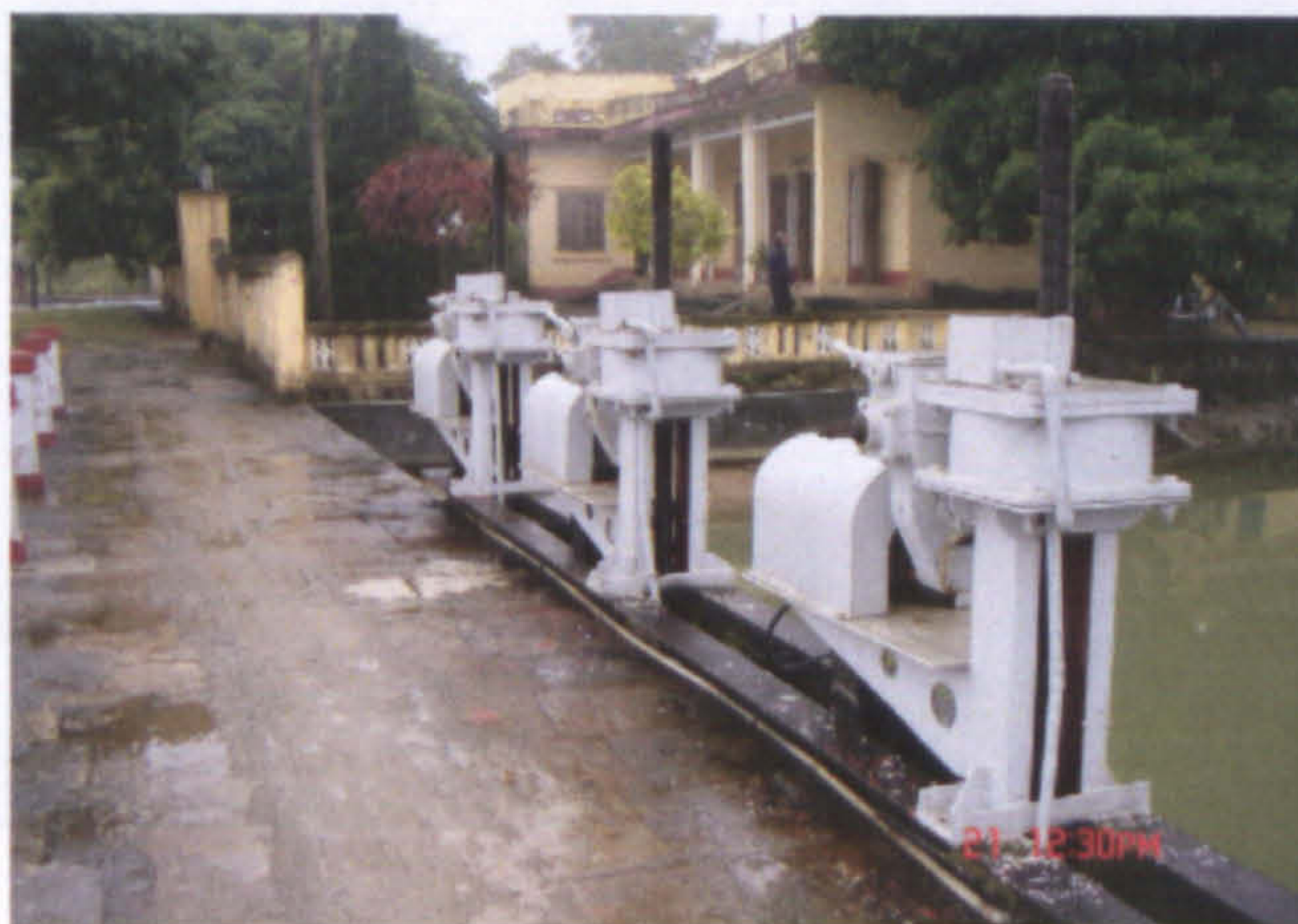
Plate 3 – Gate valves on Quy Xa Sluice
