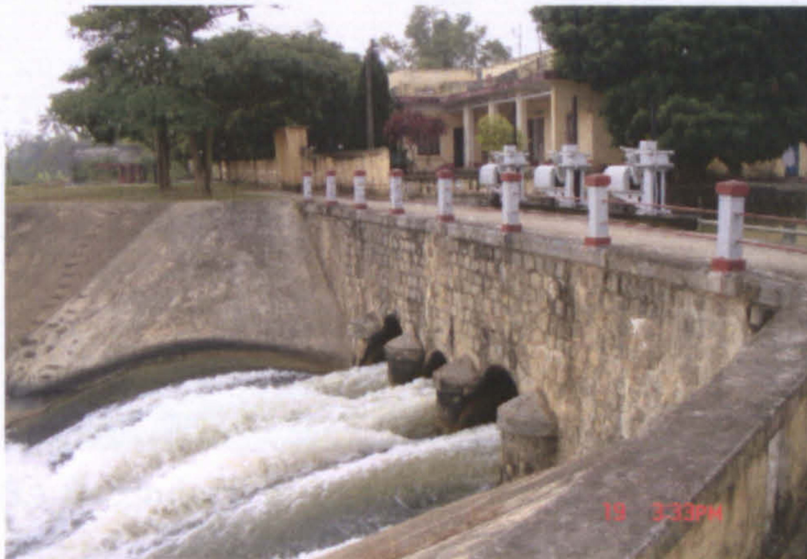
Plate 2 - Quy Xa Sluice, control water from Chu River to irrigation systems
