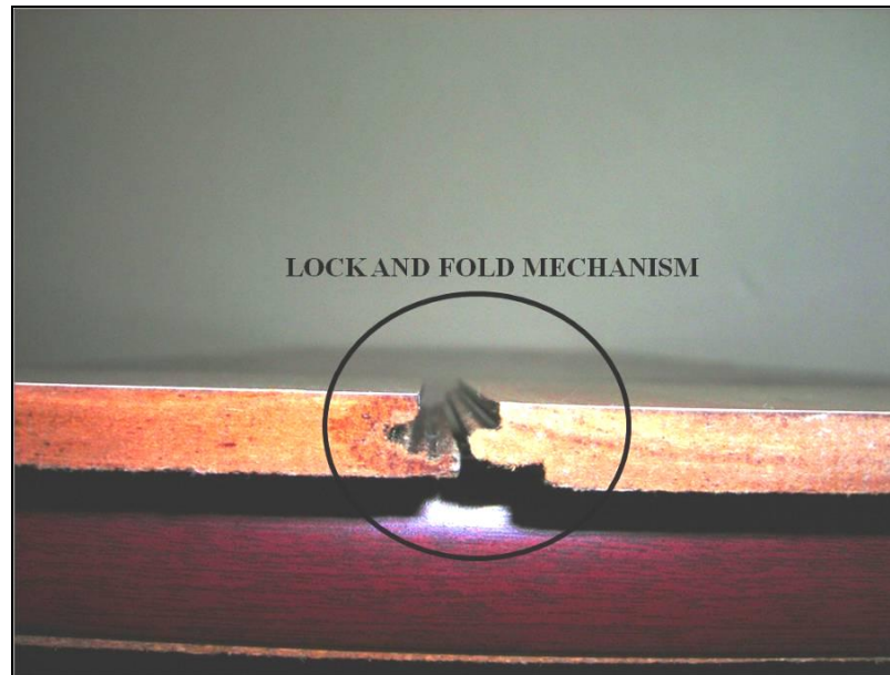
Figure 1.1: The lock and fold mechanism of the floating floors.
